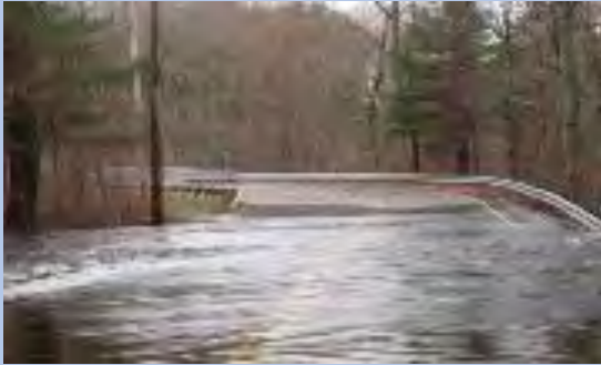
Riverine and Stormwater Flooding
