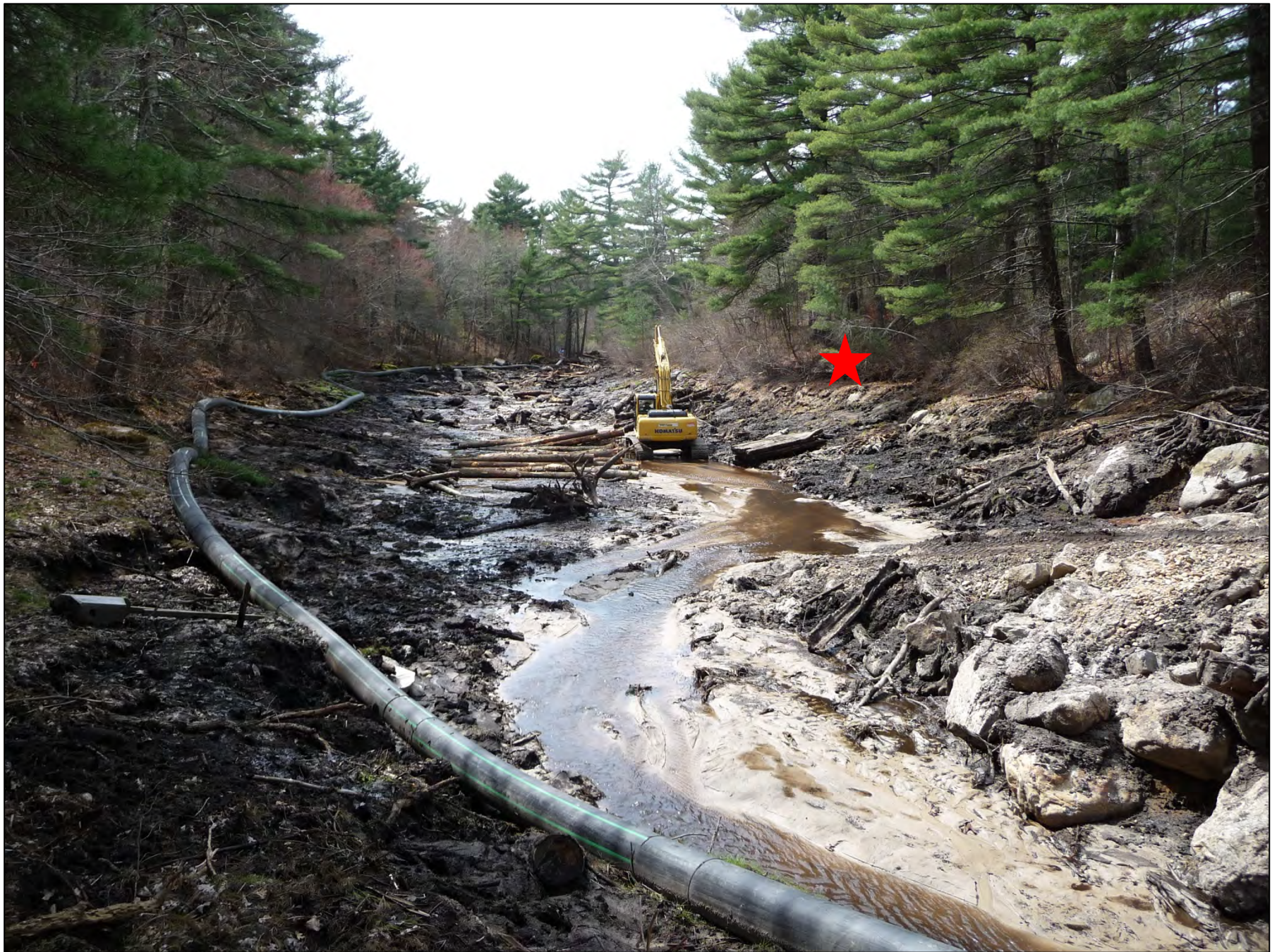
Dam removal on Eel River (Plymouth) - 2010
